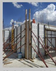
Adjust the alignment and plumb line measuring just before casting. Cast using S4 concrete (thixotropic type, max aggregate granulometry 20 mm).
