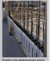
as a final result, will form a mesh consisting of horizontal and vertical rods similar to electro-welded mesh.
