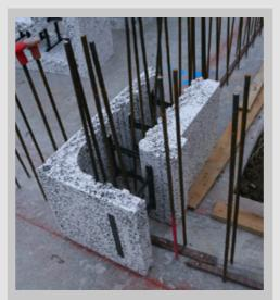
Start the first section starting from the corners and continue with the installation of the linear blocks.
