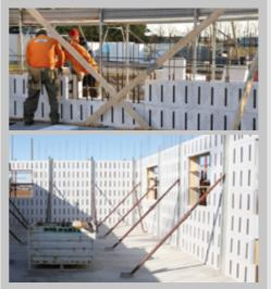
Proceed up to the envisaged height and fix the alignment and plumb line measuring system to the Climablock.
