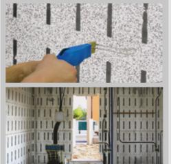
The installers autonomously mark out the area safely and quickly using a hot knife.
