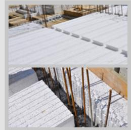
When creating the slab, the continuity of the external insulation is not interrupted, thus avoiding thermal bridges; moreover, the edge of the slab has already been made.
