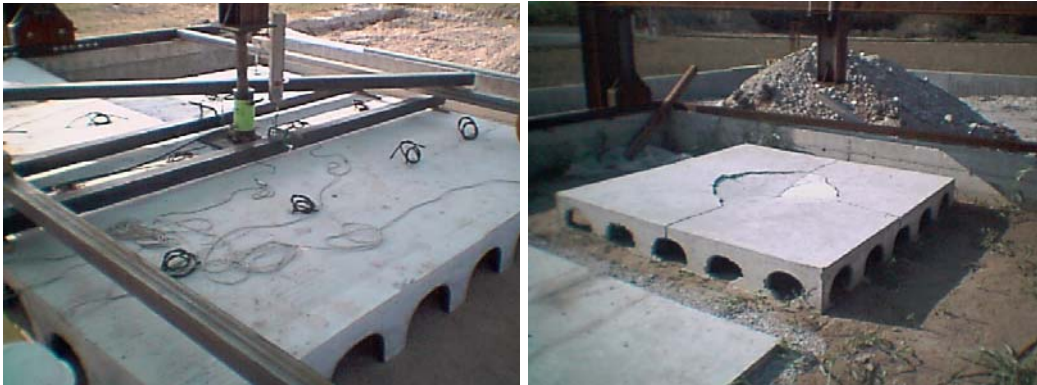
Figure 5. General view of the test tank with a) a typical pavement on PDSEs before load application and b) at the end of the test.
